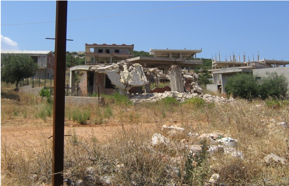
(Case demolite a Ksamil)
